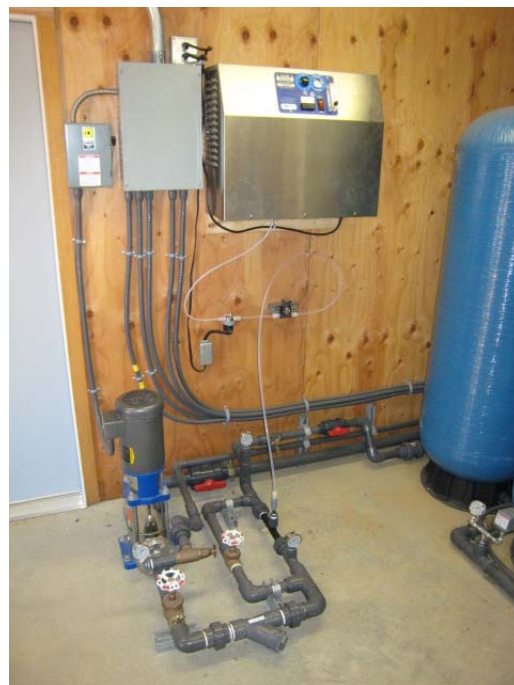
Ozone Injection System for Private Well
