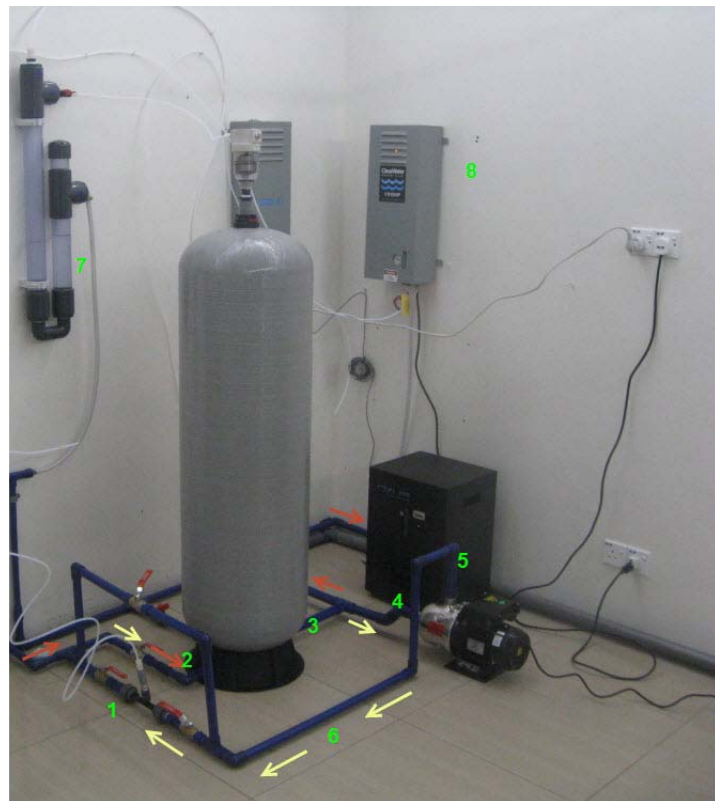
Recirculating Pressurize Contact Tank Ozone Injection System
