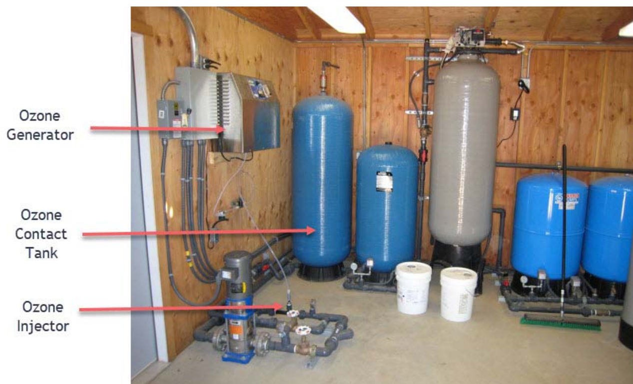
Single pass ozone injection with large oxygen-fed ozone generator and contact tank.
